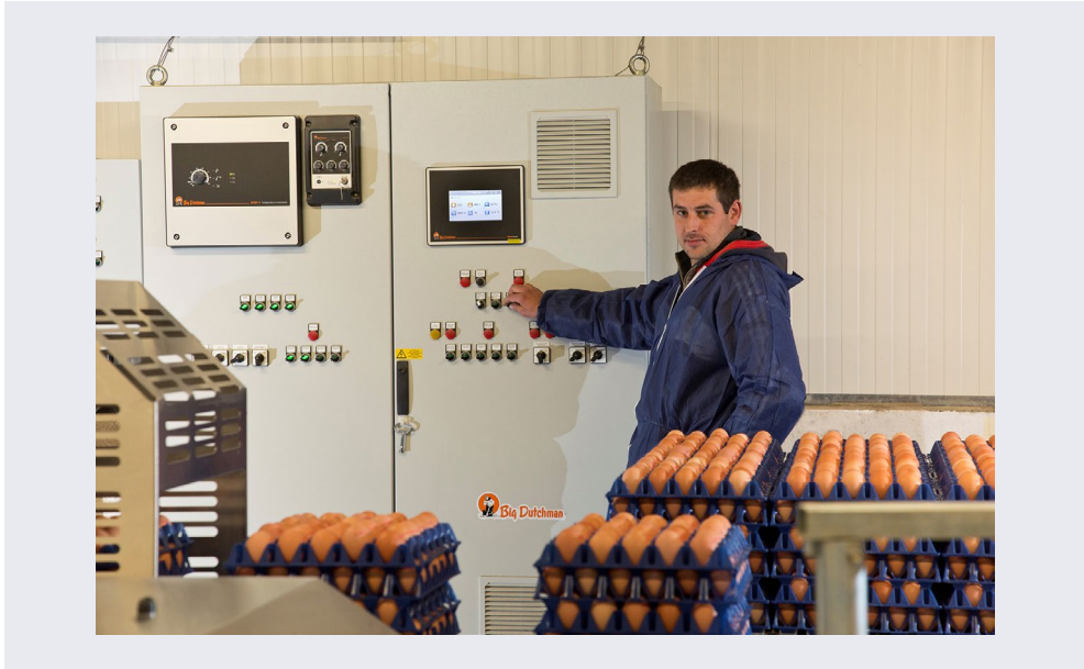
Figure 10.2. Transfer of Technology through the medium of provision of equipment. Control units can regulate livestock house environments by operating ventilation, temperature and humidity controls in response to data received from sensors in the animal environment. Similar control units can deliver measured quantities of diet ingredients to livestock according to pre-determined algorithms. The incorporation of contemporary best-practice knowledge within automated systems offers to livestock managers the benefit of one-step Technology Transfer mechanisms (image: Glenrath Farms).
